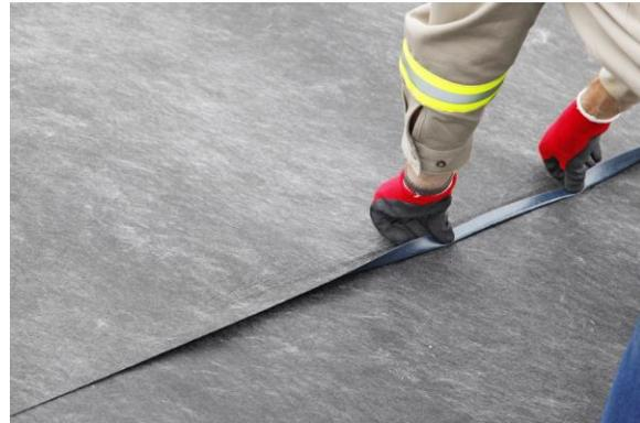
**NOTE:** The liner sections must all be unrolled in the same direction in order to keep the gray/black and colored tabs properly aligned.
