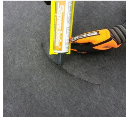
10.1.4. Once a tear is repaired from the bottom, proceed to patch it as stated in sections 10.1.5. – 10.1.13.
