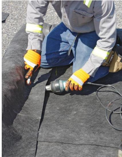
11.2.3.4. It is recommended to have a 6" to 8" welding tab. To prevent the foam from shifting, this tab must be completely welded.
