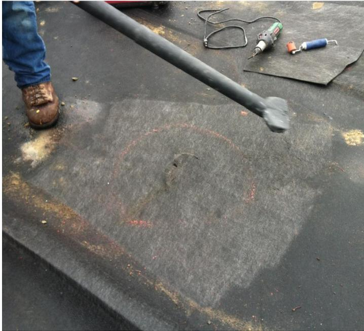
10.1.3. To prepare fork tears for patching, place a piece of liner underneath the tear to reinforce the area. Use the hot air gun to tack the reinforcement layer and liner together. This gives strength to the damaged area. Force SilapreneSolidSeal<sup>®</sup> sealant along the edge of the tear.
