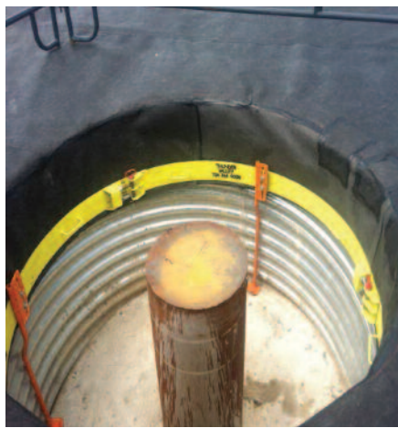
The liner should be attached to the cellar walls, either mechanically or with a coating, to prevent any backup at the wellhead from pushing under the liner. Cellar attachment options pictured here are, clockwise from top left, an ice guard, spray urea, cementing the liner column, and metal ring.
