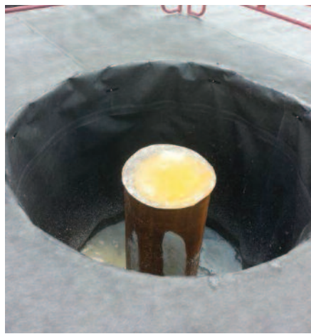
The liner should be attached to the cellar walls, either mechanically or with a coating, to prevent any backup at the wellhead from pushing under the liner. Cellar attachment options pictured here are, clockwise from top left, an ice guard, spray urea, cementing the liner column, and metal ring.
